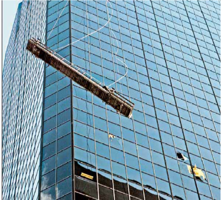
A gondola strikes a building after being violently blown by the wind in Denver, Colorado (2005/12/01 NHK News).
